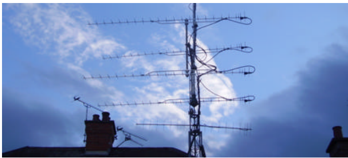
G8VHI's new 4 x23 el Wimo yagi array
