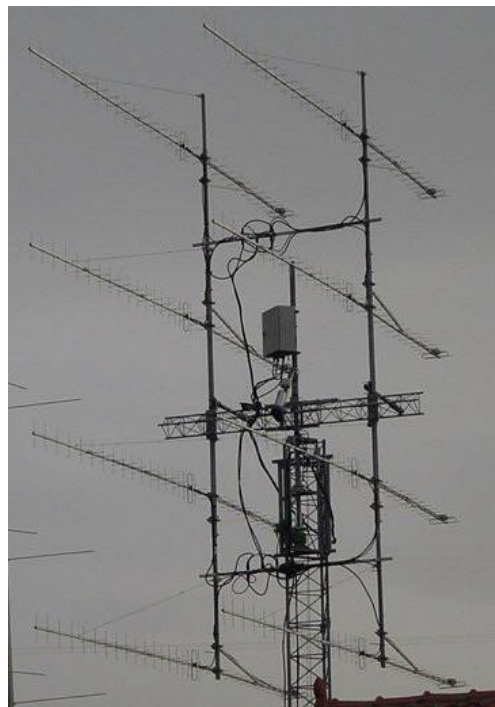
SV1BTR's new 70cm cross yagi array
