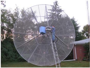
Installing 10 GHz system for K1JT operation
