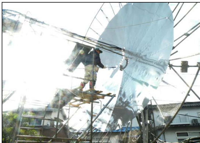
JA4BLC is preparing for the EWW microwave contests by covering the center of his dish with solid AL foil.
