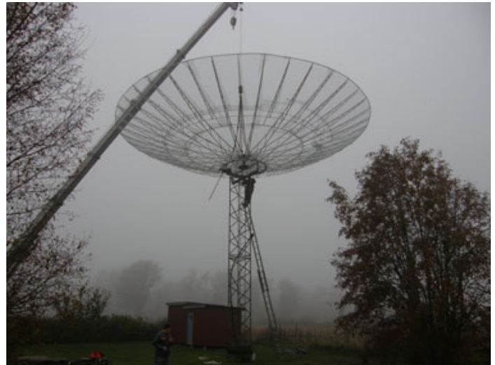
SM4IVE's new 13 m dish going into place
