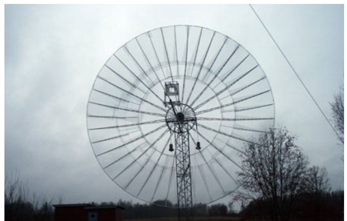
Dish with feed pole and mounts in place
