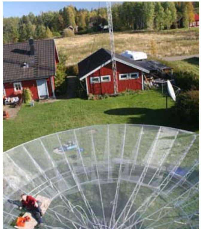
Lars putting the surface on the dish
