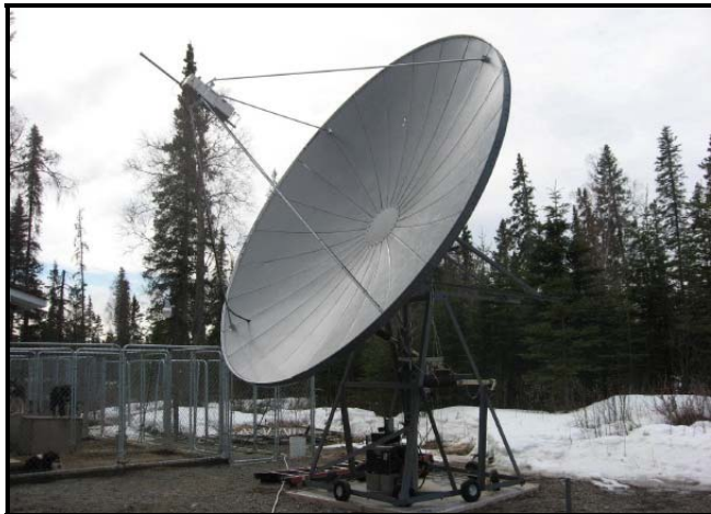
KL6UW's new 4.9 m dish with 70 cm quad feed in front of 23 cm horn
