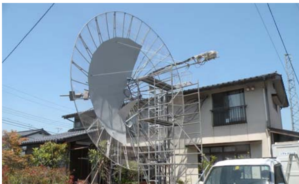
Removing aluminum foil surface from JA4BLC's dish
