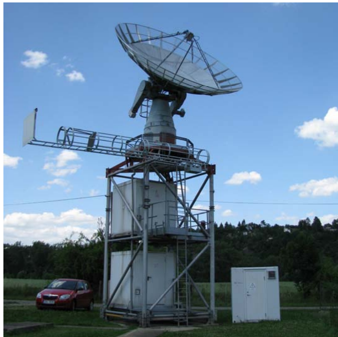
New extended 6.4 m dish at OK1KIR
