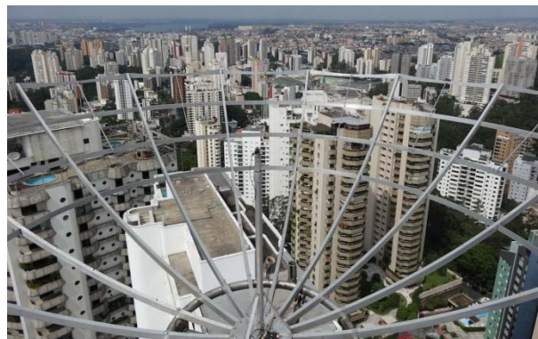
View from PY2BS's new dish while under construction
