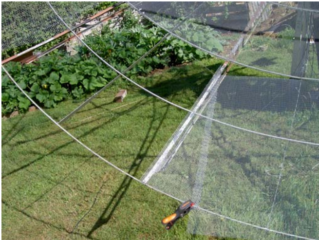
New mesh being installed on G3LTF's 6 m dish
