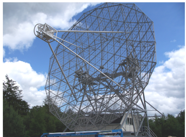
New (renovated) PI9CAM 25 m dish
