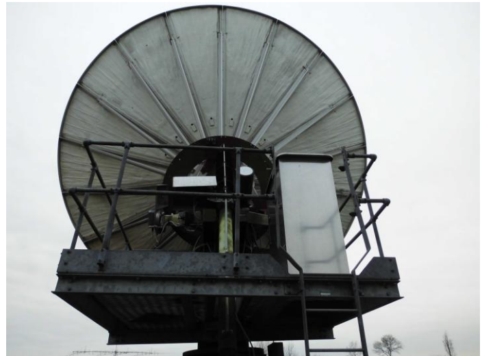
Another view of DL0SHF's 10 GHz EME beacon 7.8 m dish
