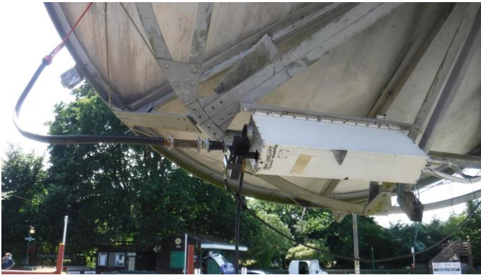
G4RFR's new TWT mounted behind their dish
