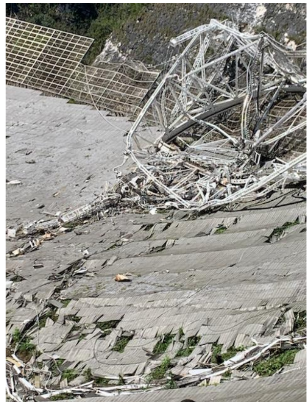
Collapsed Arecibo - credits: https://www.nsf.gov
