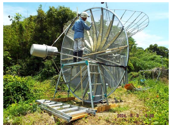
Figure 30 - JA6AHB dish repair
