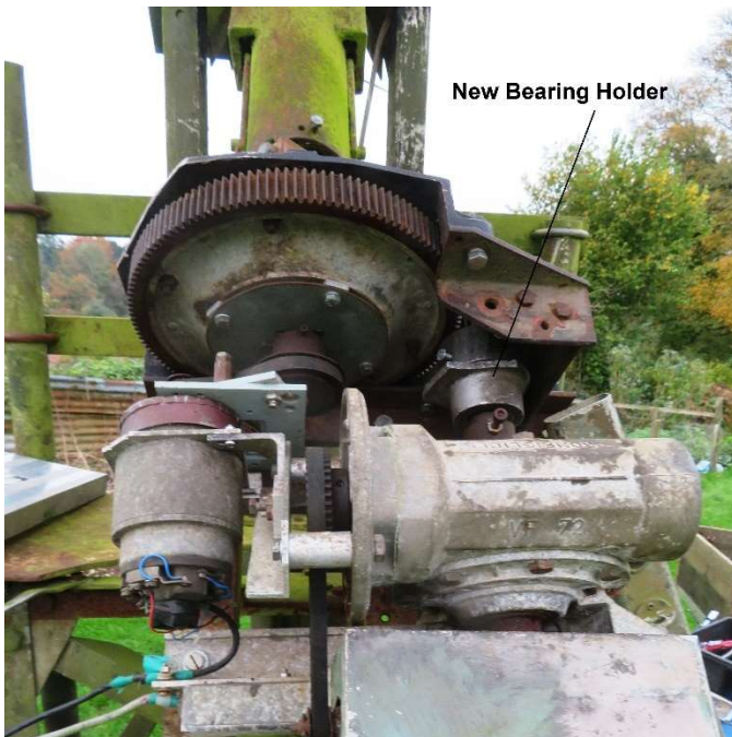
G3LTF Repaired Hour Angle Drive
