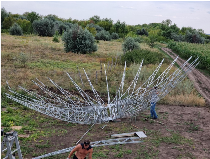
RD4D 10 m dish rib assembly
