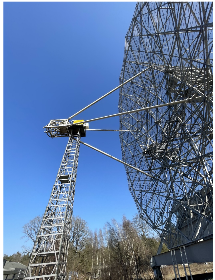
PI9RD dish maintenance position
