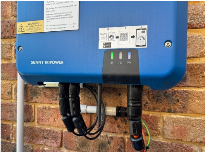
VK2CMP Ferrite Installation on Solar Inverter
