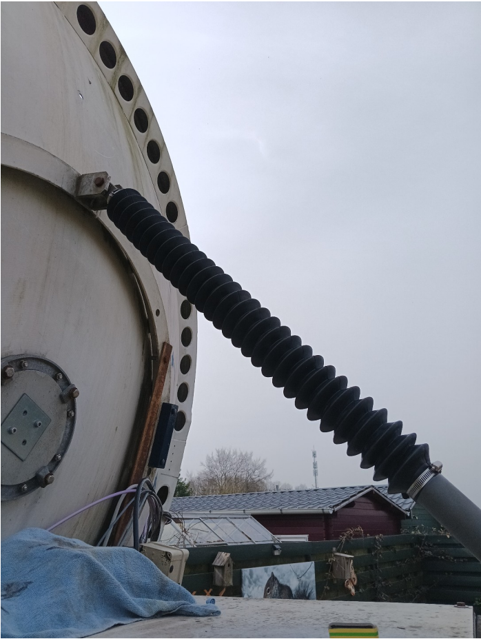
PAOPLY Replacement Boot Installed
