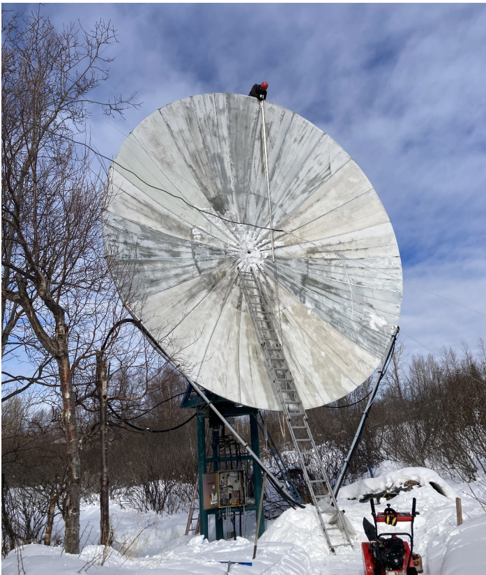
KL6M Dish Repair Work
