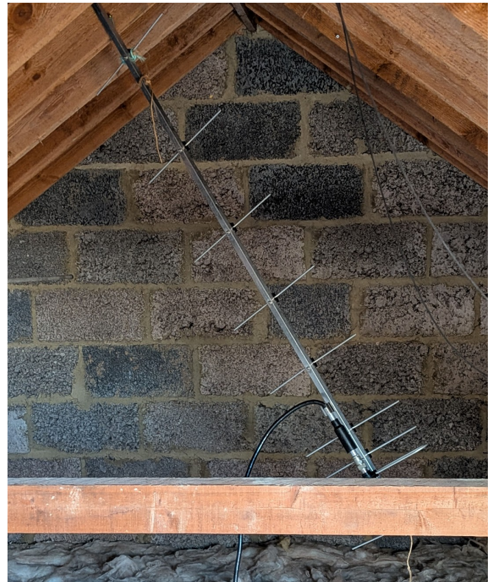
G3YEG 9-element Yagi in Attic
