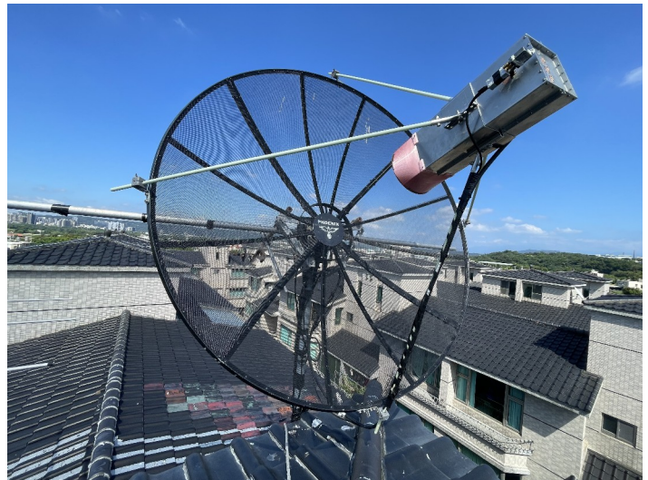
BV3CE 1.8 m mesh dish CP feed 200 mm flare
